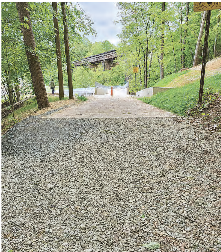
Looking north down on the new bridge.
