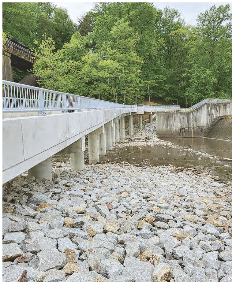
The new bridge clears the spillway.
